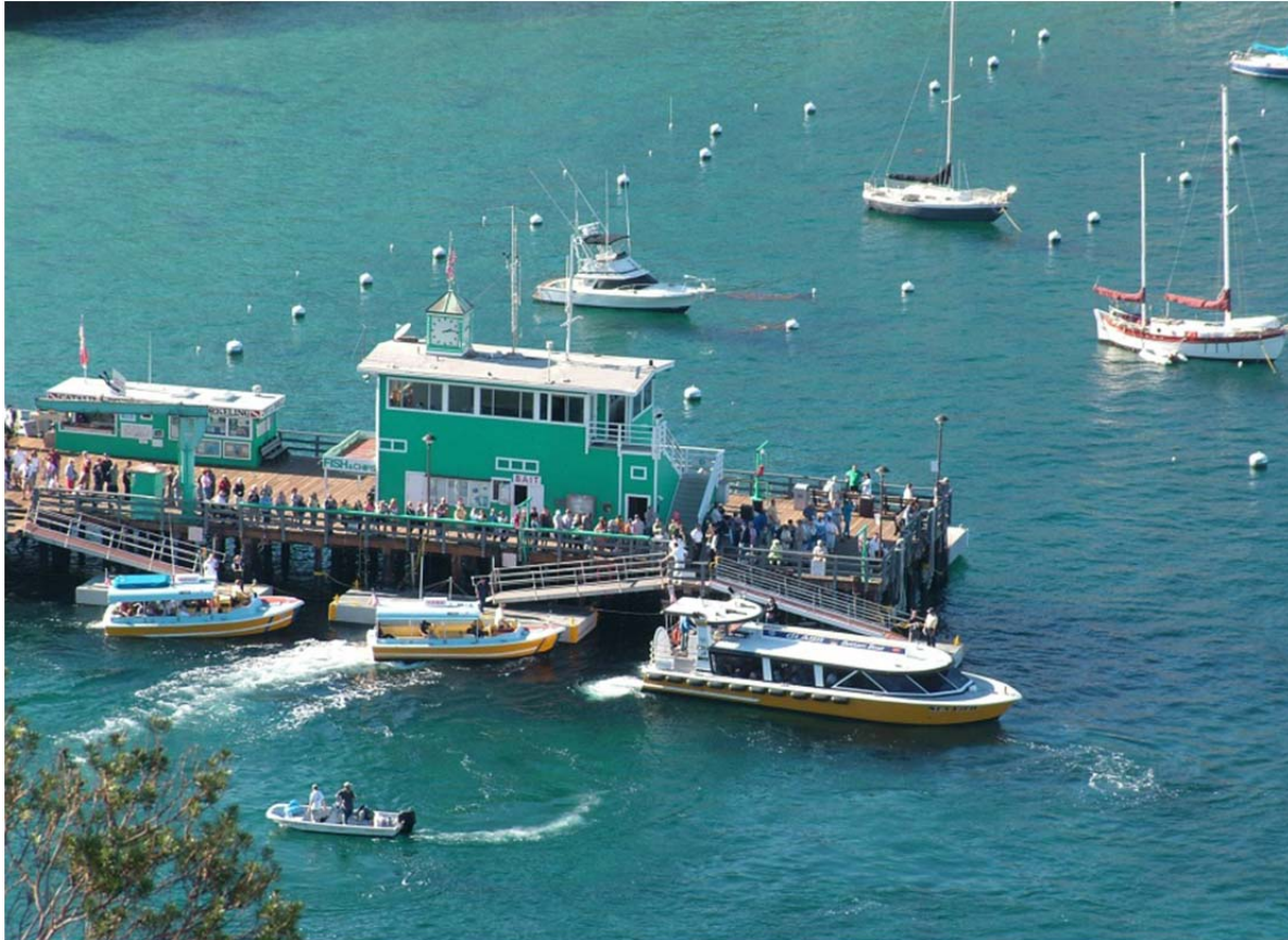
Winter Floating Dock Operations from the side of Avalon Pier
